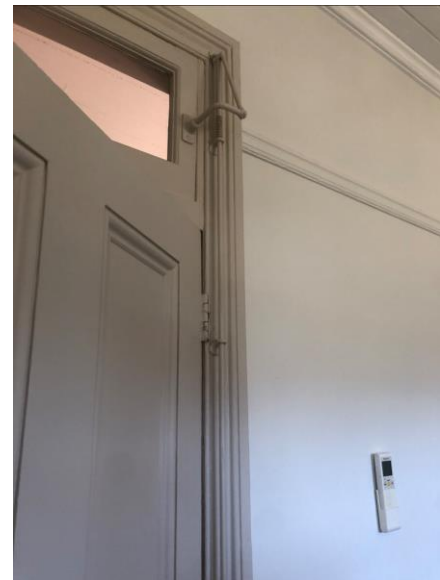
Figure 21: Door details with transom window, cover moulding and traditional door hardware in Ranger's Residence.
