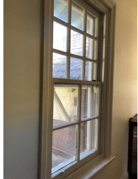
Figure 23: Multi-paned, single-hung window details at Ranger's Residence.
